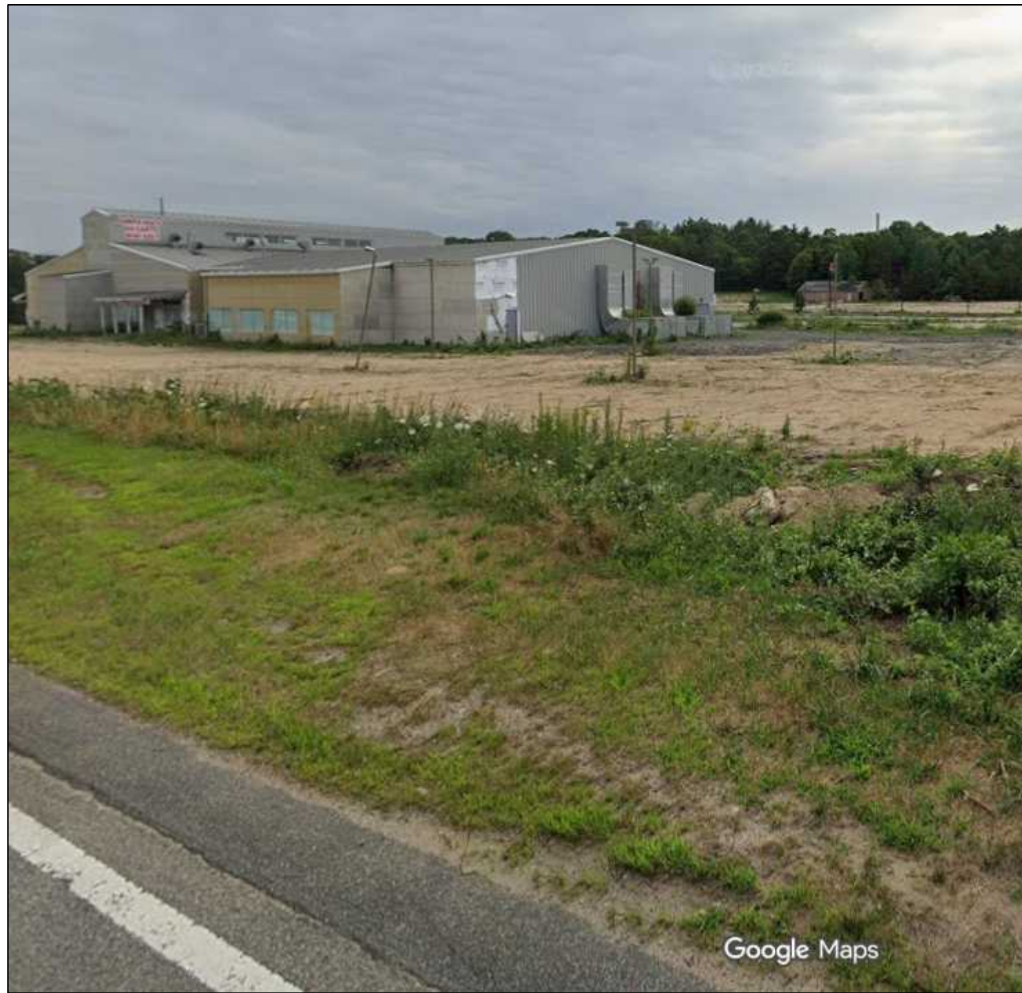
Existing View Southwest to Site from Southbound Roadway
